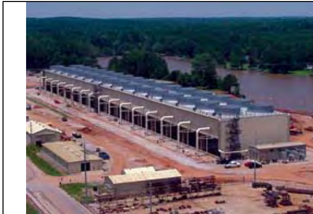
36-cell, space saving back-to-back inline conventional cooling tower. From: GEA Power Cooling Systems website
