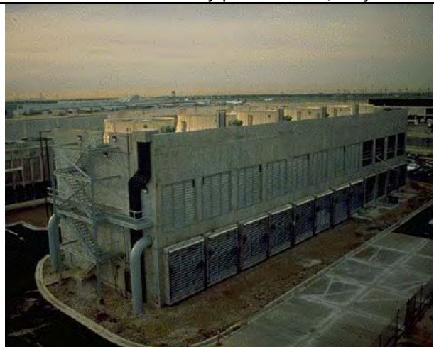
Operational plume-abated tower, ~50 ft. tall – Chicago O'Hare Airport Source: P. Lindahl – Marley presentation, May 2002.
